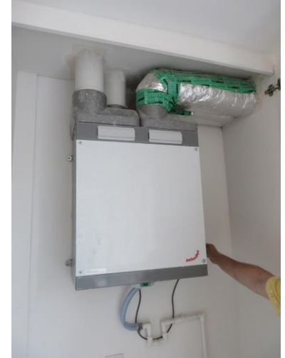
Heat Recovery Ventilation (Communal room unit)
