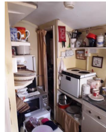
Cramped like Kitchen conditions with no extract and serious condensation formed during cooking (62 yr old kitchen)
